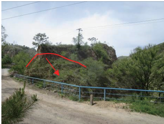
Figure 3 Small slump of the north slope side
